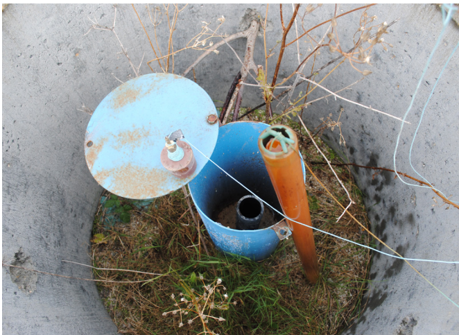
BH 204 – inside manhole ring
