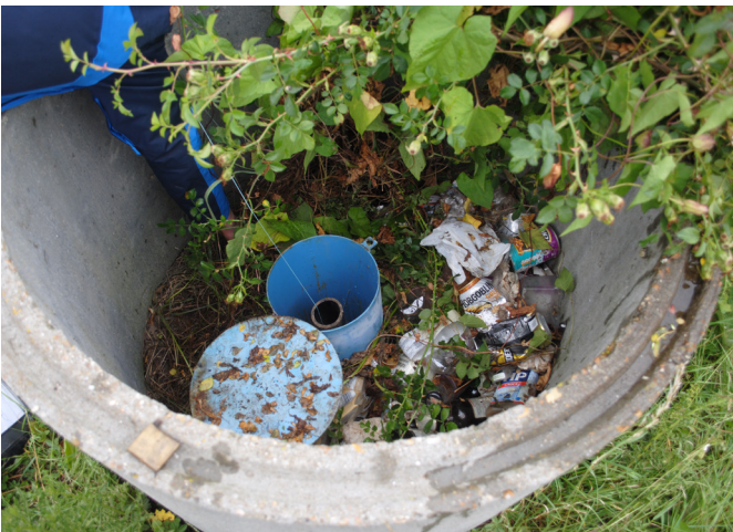
BH 707 – inside manhole ring
